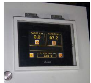
Advanced Operation Panel with Remote Display and 4-20 mA Analog Outputs
