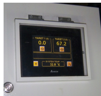
Advanced Operation Panel with Remote Display and 4-20 mA Analog Outputs
